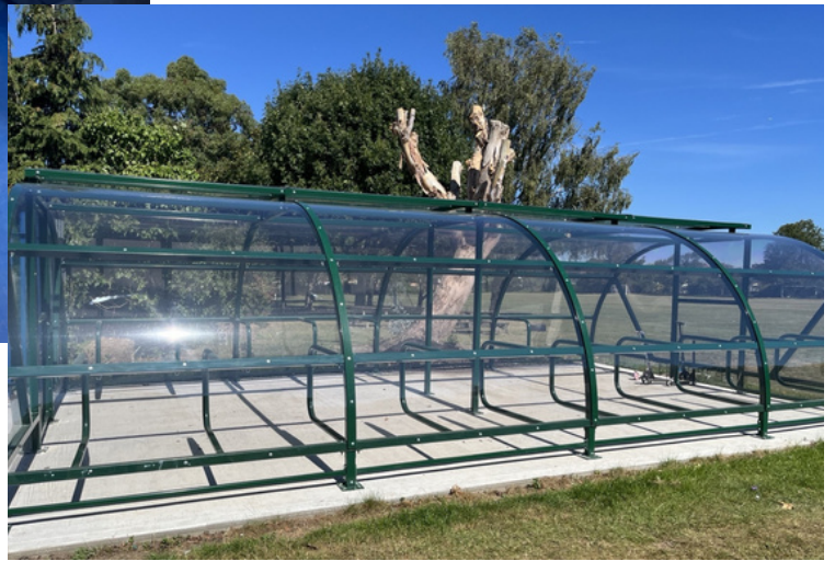
The new bike shed
